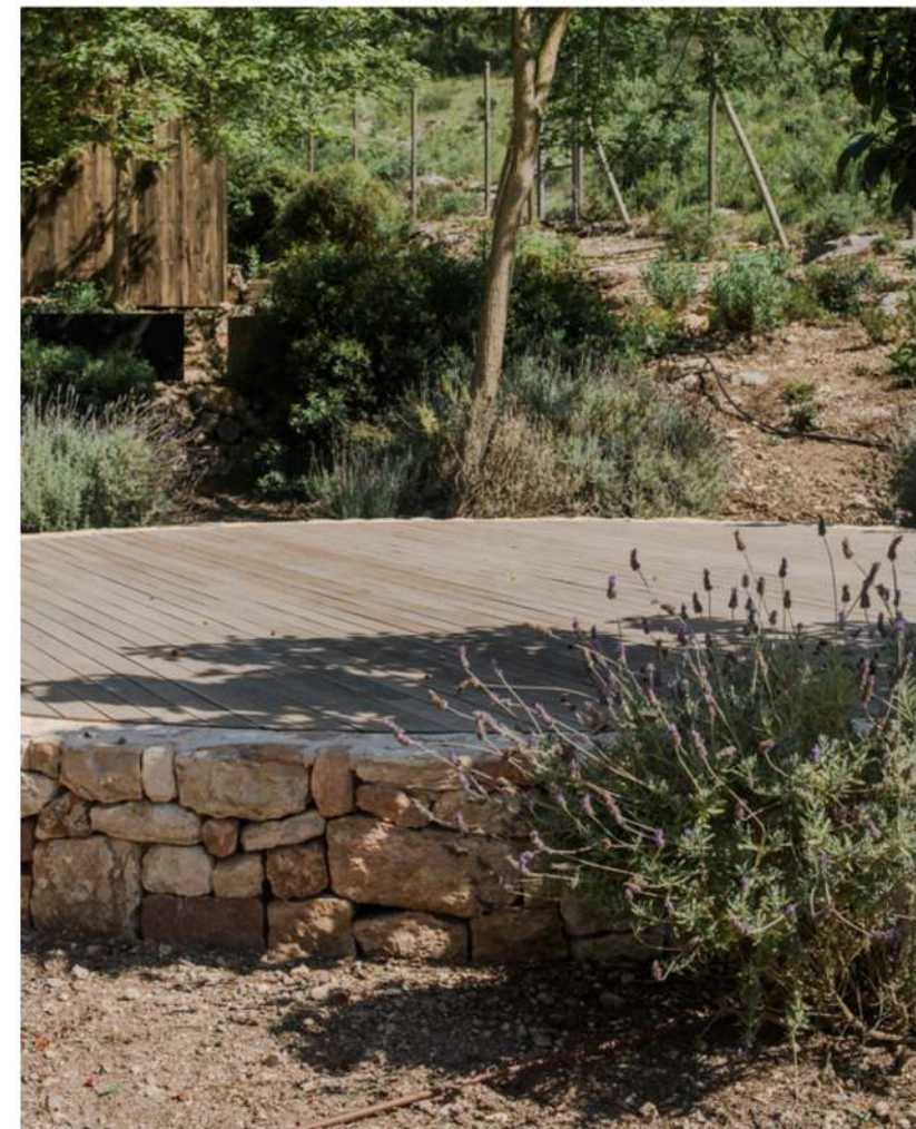
dry stone base with wooden decking and vegetation around or aromatic herbs
